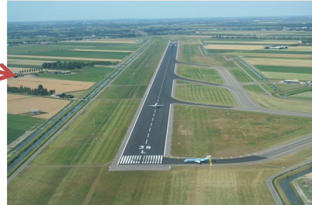
b) Airport Runways
